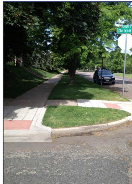
7th Avenue curb turf restored
