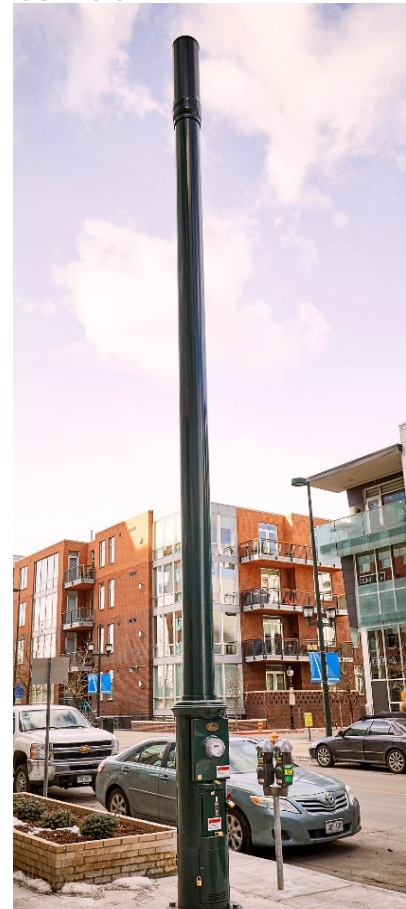
Figure 5-1: Freestanding Small Cell Pole
