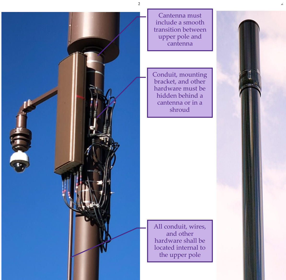
Figure 5-3: Acceptable Type 4 Installation
