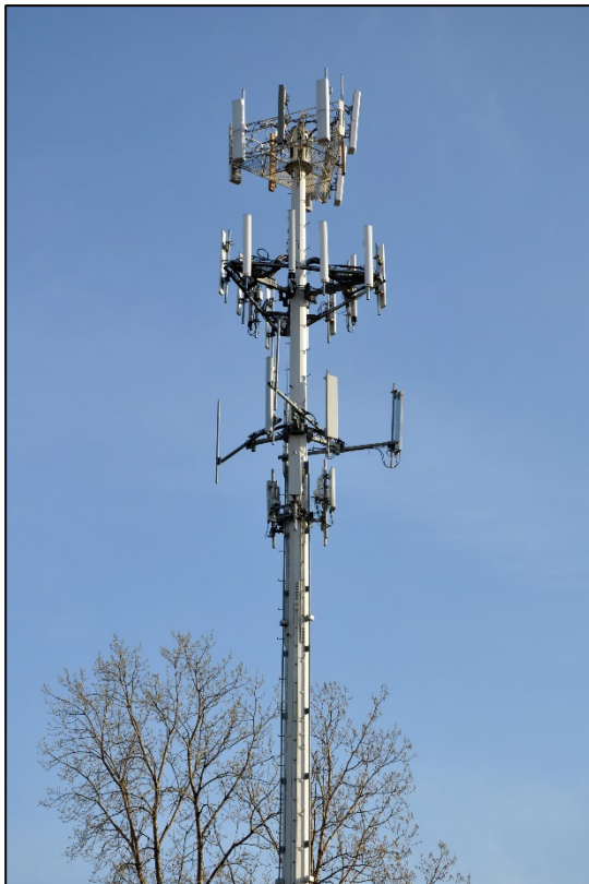
Typical large cellular antenna.
