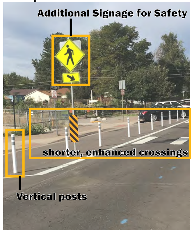
Safety improvements at E 13th Avenue at Xenia Street.
