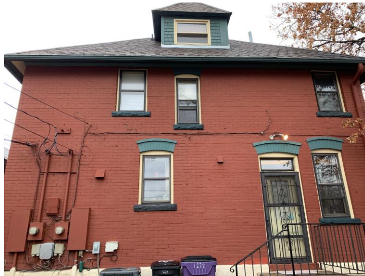
Photo 3: East facade, Winter 2020
