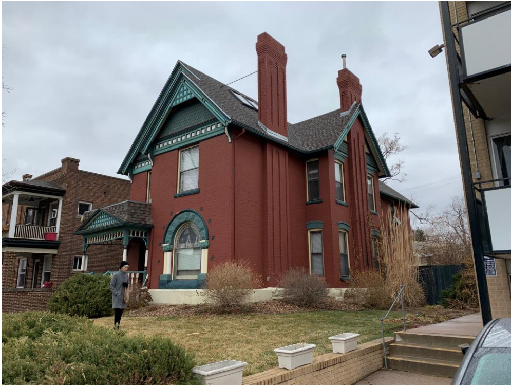
Photo 1: 1272 N Columbine St., Southwest façade, looking northeast, Winter 2020
