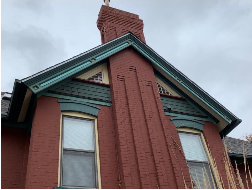
Photo 7: Chimney detail on south facade, Winter 2020
