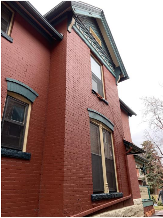
Photo 5: North façade, looking southwest, Winter 2020
