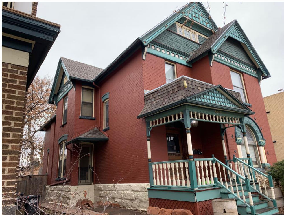
Photo 2: Northwest façade, looking southeast, Winter 2020
