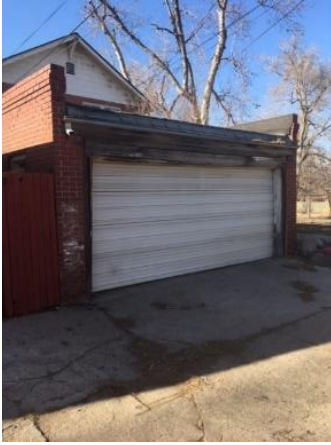
780 Steele St, Garage (non-contributing)
